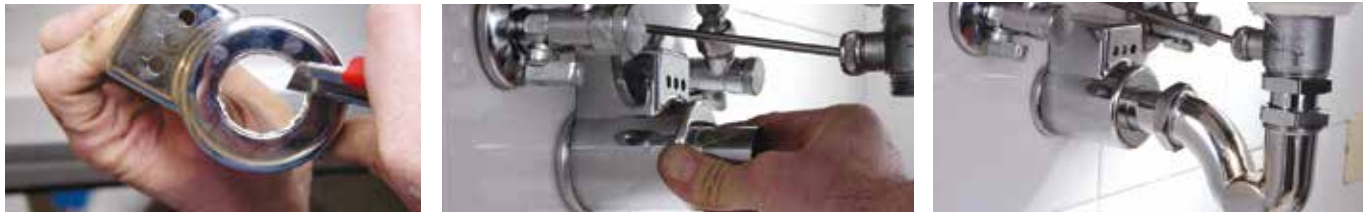
5. Fix the chromed cover 6. Connect the trap
