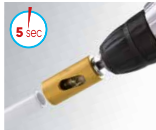
2- Chamfering the pipe
