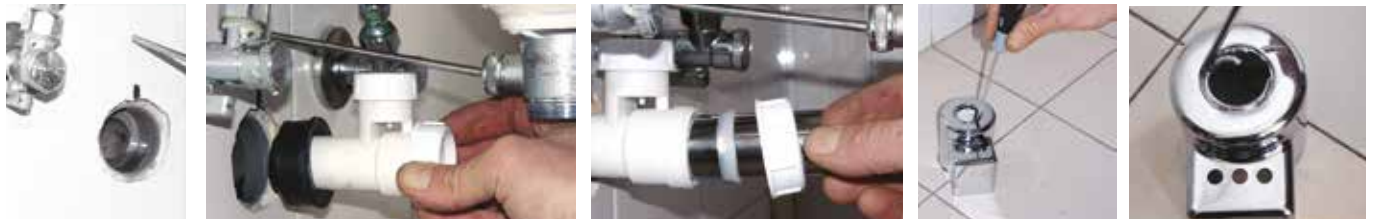
1. Remove the trap 2. Install the AAV with technical gasket 3. Connection with chromed pipe 4. Create the correct space to connect the trap
